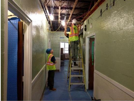
... while Fraser (the HVAC subcontractor) began removing the steam radiators and installing hangers for the new hot water pipes to service the new radiators.
