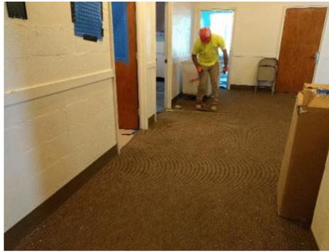
Following behind the demolition work, the crews have been isolating and removing exposed asbestos as it is encountered. At this point, they have abated a substantial portion of the first and second floors.
