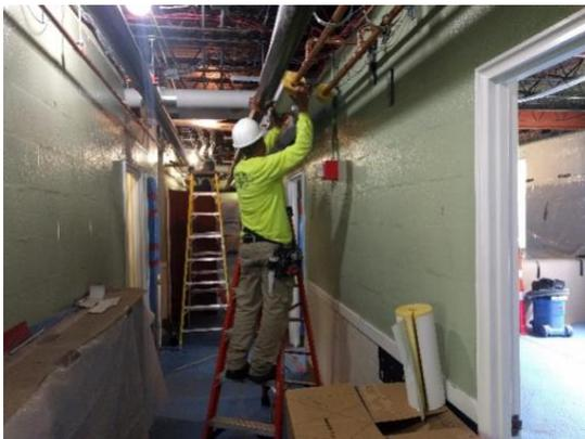
In addition, Fraser, the HVAC subcontractor, has been insulating the hot water pipes on this floor.
